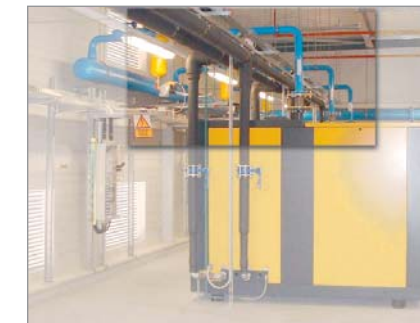
Fig. 3b: Vibration-dampening compressor connection with axial compensators
