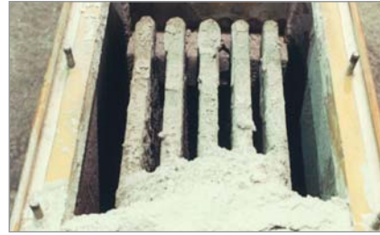
Fig. 2a: Bag air filter (intake side)
